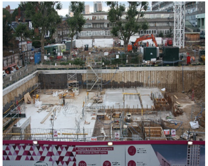
Plot 18 progress on site
