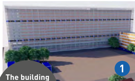
1 The building is wrapped in monarflex sheeting.
