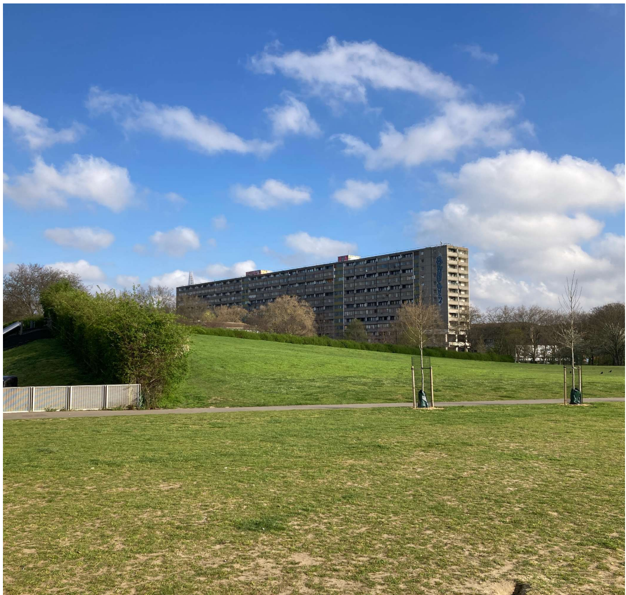
Figure 9: Aylesbury Estate, view from Burgess Park
