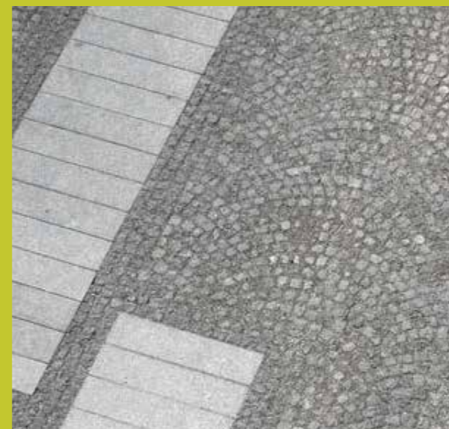
Paving cubes laid in 'Venetian Fan' pattern
