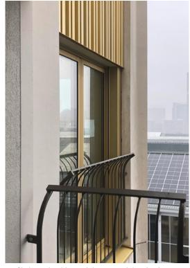
Profiled panels add visual density and detail. Edges are held with refined flashings, and fixings are hidden.
