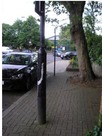
L25 – Reduction of the effective width: non-aligned obstructions
