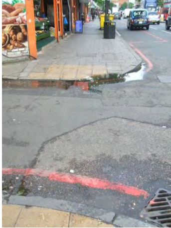
C4 – Lack of consistency of the surface and drainage issue
