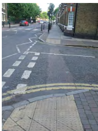
C40 – Poor surface quality due to inadequate reinstatement of materials
