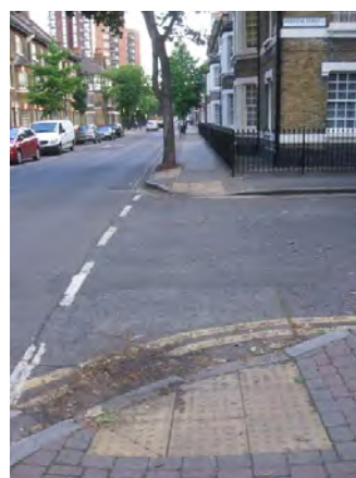
C41 – Poor surface quality due to lack of maintenance
