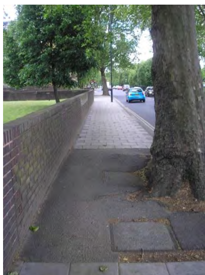
L29 – Past use of inappropriate materials and gaps/undulations due to tree root growth
