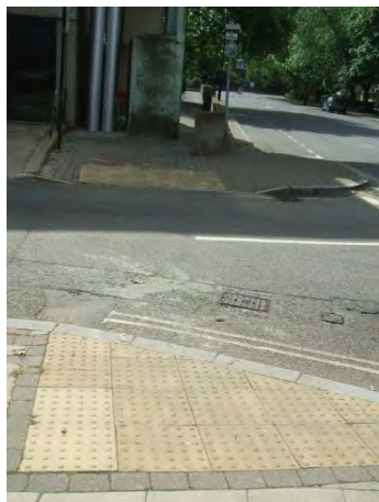
C47 – Poor surface quality due to inadequate reinstatement of materials
