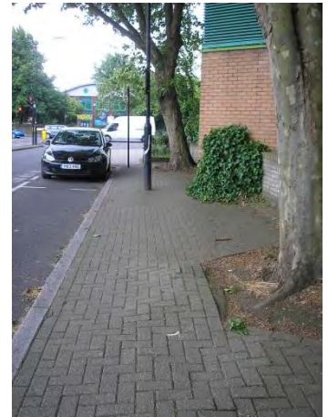
L25 – Undulations/gaps due to tree root growth
