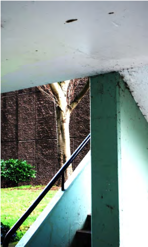
Image 2 – Basal stem of retained tree T41 showing proximity to building and levels. Protection prior to any on site demolition is required to successfully retain this tree
