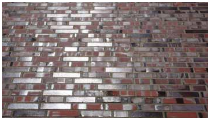
Fig 5.7.2 Semi-glazed clinkers have lots of visual interest and catch the light- good for tall build-
