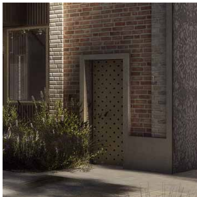
Fig 5.12.22 Secondary metallic entry doors in aluminium.
